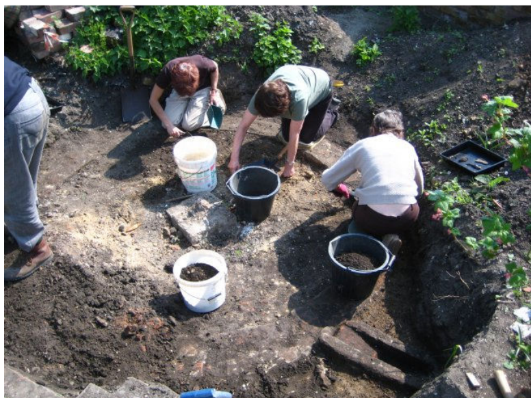
Fig 2. Work begins to reveal the structure.
