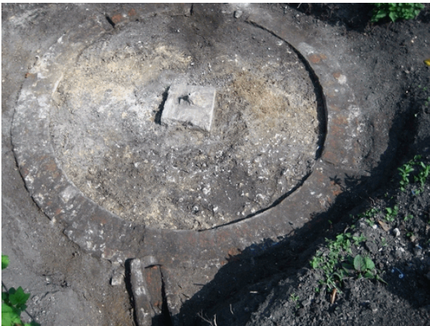
Fig 3. With the first context removed the complete structure was revealed.
