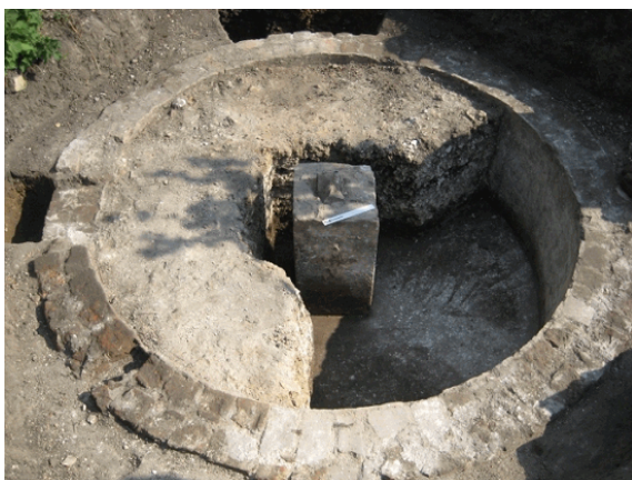
Fig 9. Revealing the lead pipe.
